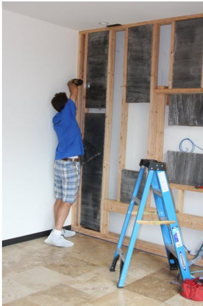
The above image shows us installing the carbon into the stud spaces of a recording studio wall.
